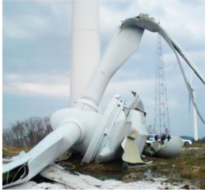
Fig. 2: Turbine part on the ground
